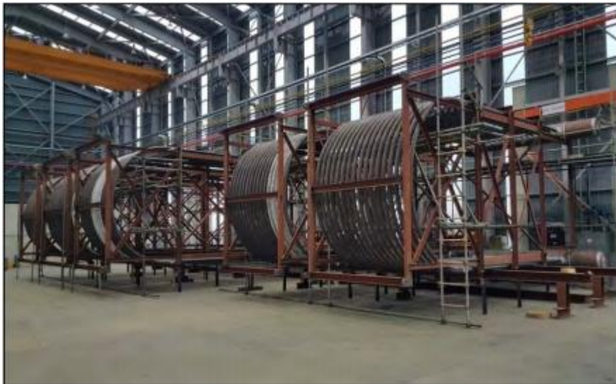
RADIANT ABOR COIL WELDING
