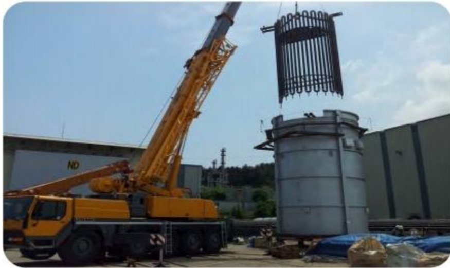
RADIANT MODULING
