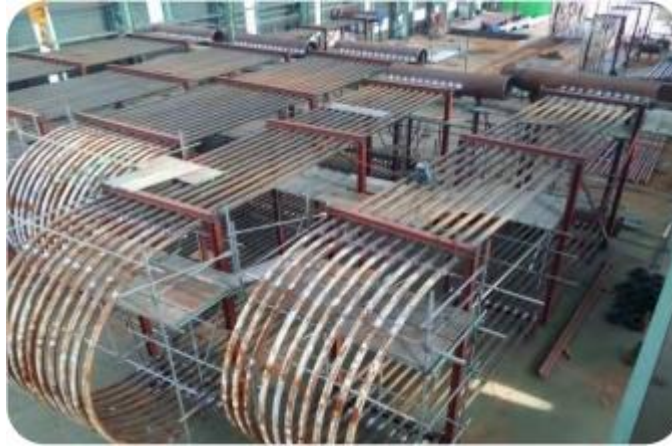
ARBOR COIL WELDING
