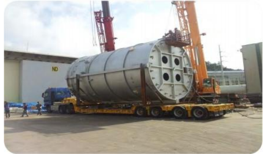
RADIANT MODULE TRANSPORTATION
