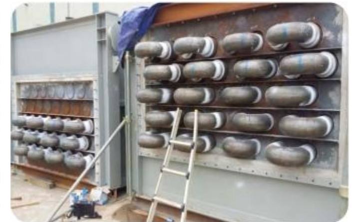
CONV. COIL WELDING
