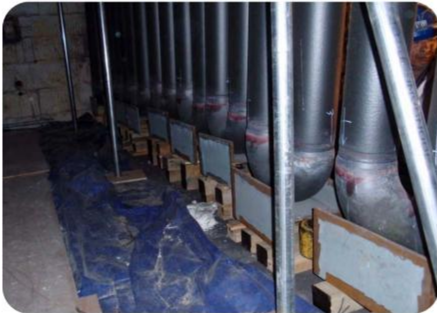
Radiant Coil Replacement
