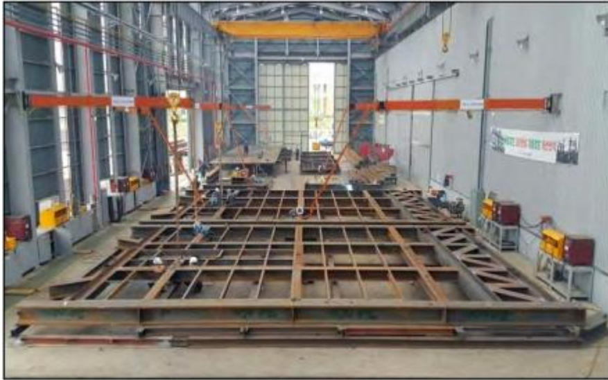
RADIANT SIDE PANEL FIT-UP & WELDING
