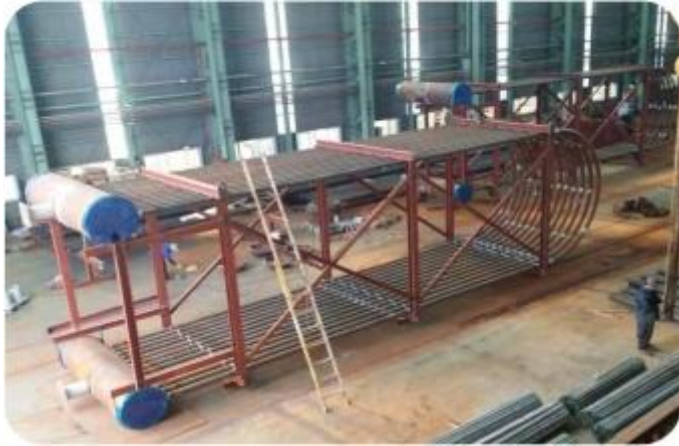
ARBOR COIL WELDING
