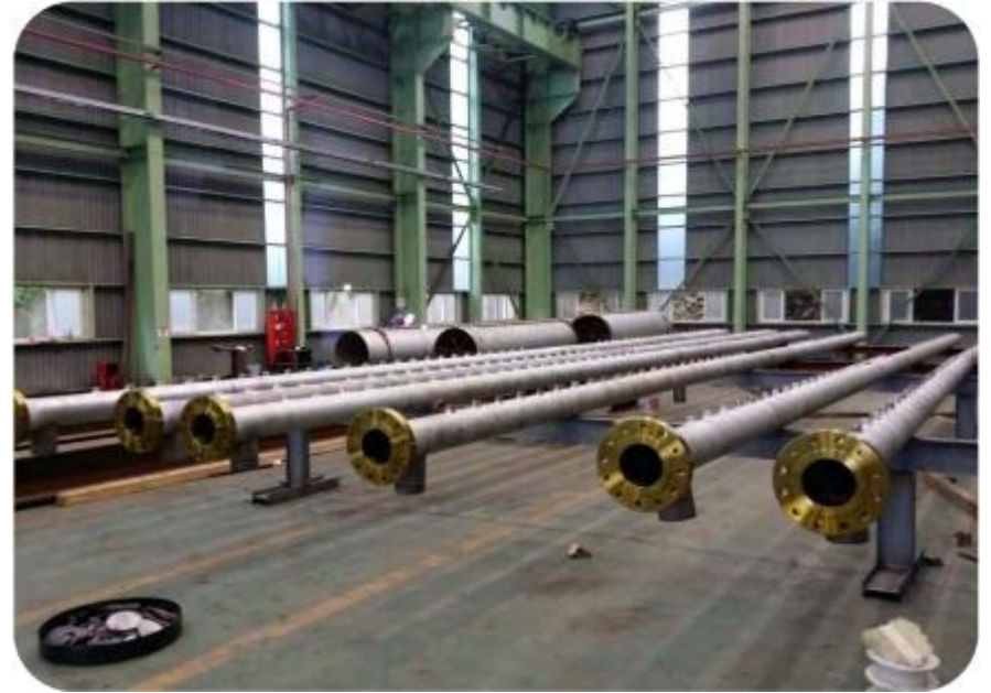
INLET HEADER WELDING
