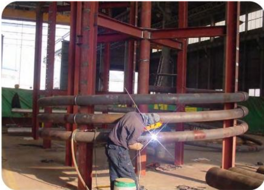
HERICAL COIL WELDING
