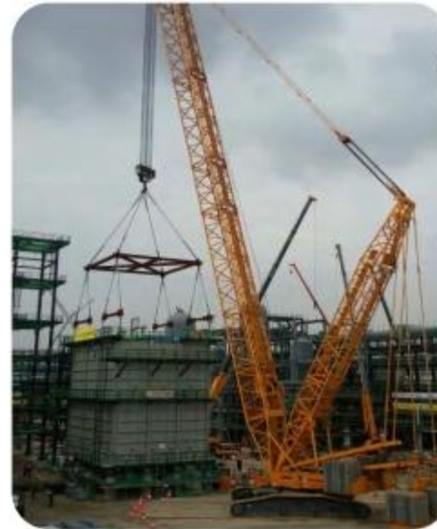
RADIANT ERECTION
