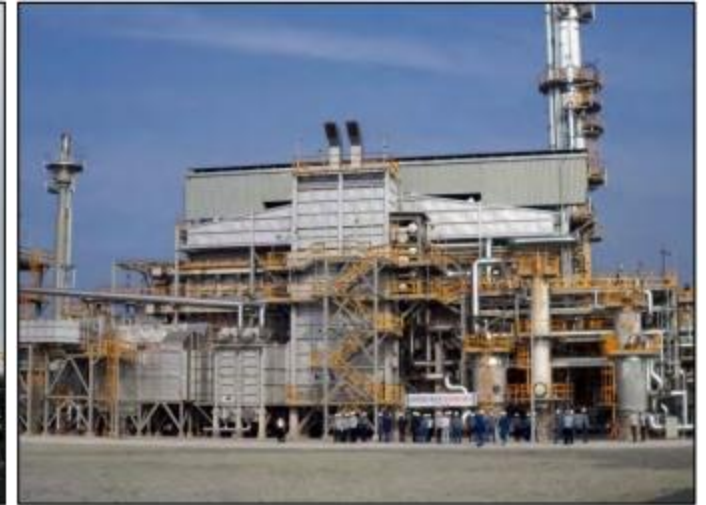
DY REFORMER PROJECT (2013) / DEOKYANG ERECTION OF STEAM REFORMER
