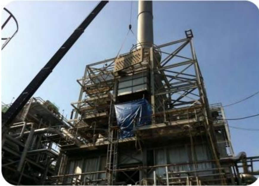
Heater Conv. Module ETS Replacement
