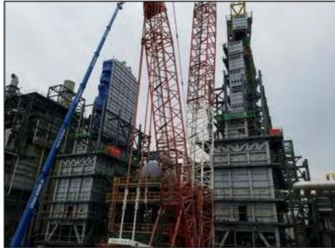
KPIC ONE PROJECT (2016) / KPIC FAB. & ERECTION OF 2 ETHYLENE CRACKING HEATER
