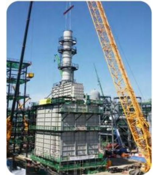
CONVECTION & STACK ERECTION
