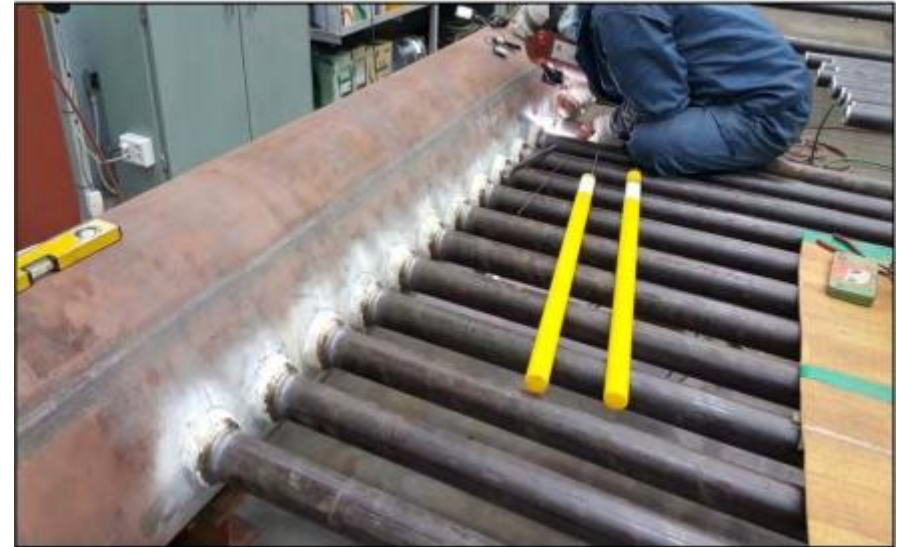
RADIANT ABOR COIL WELDING
