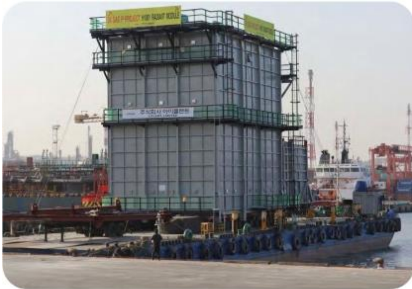
RADIANT & CONVECTION MODULE TRANSPORTATION
