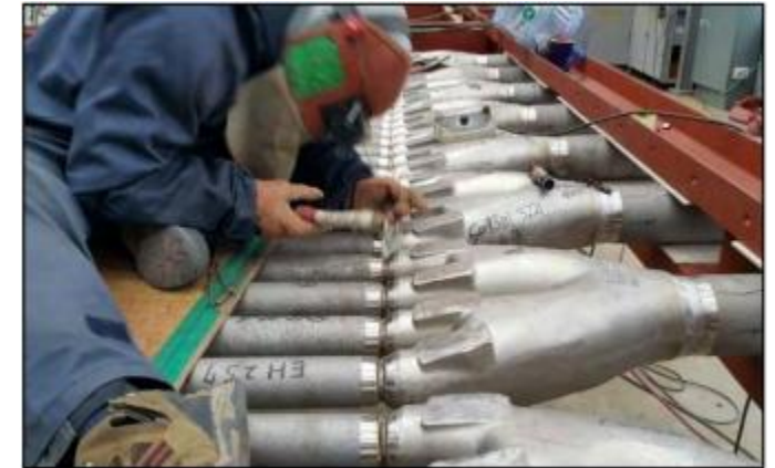
TETRA FITTING WELDING
