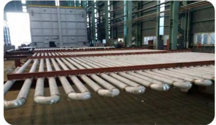
RADIANT COIL ABRICATION
