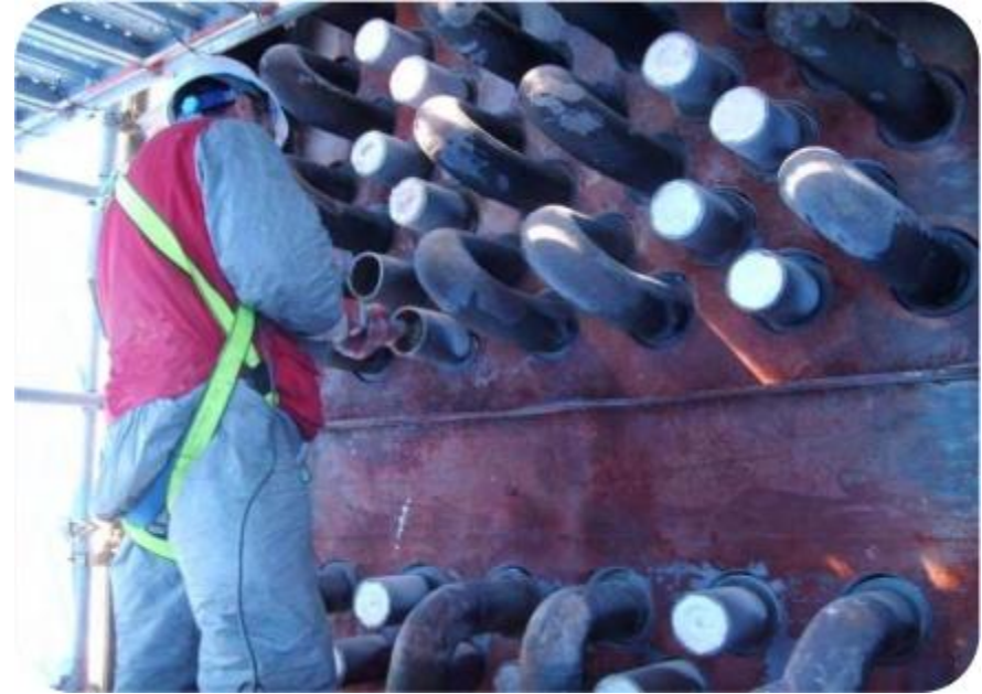
Heater Conv. Module Coil Replacement
