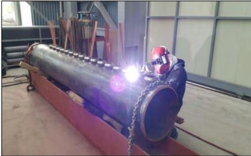
WELDOLET WELDING FOR ABOR COIL HEADER
