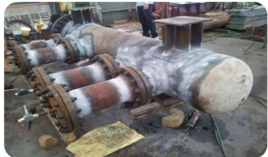
RADIANT OUTLET MANIFOLD FABRICATION
