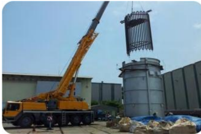
RADIANT COIL MODULING
