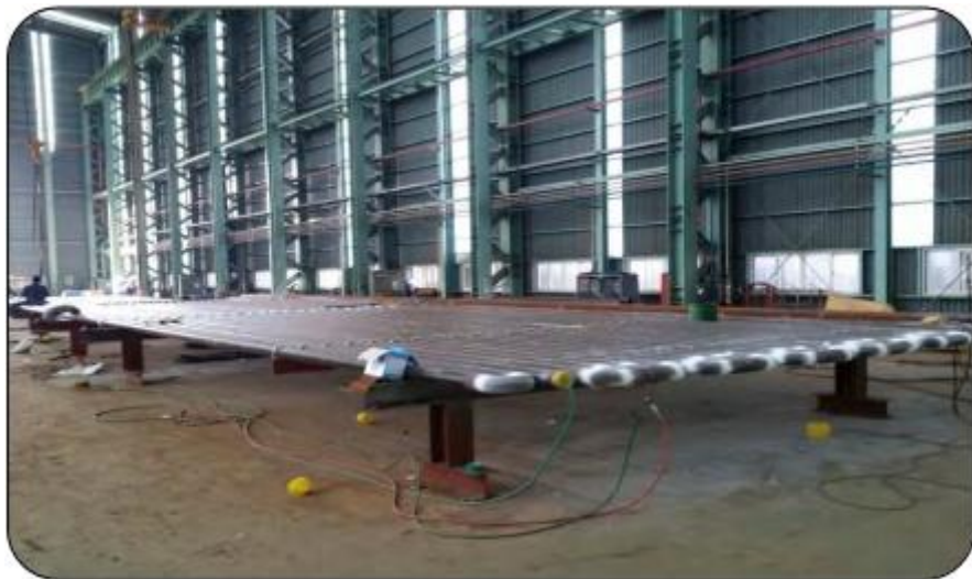
RADIANT COIL FABRICATION
